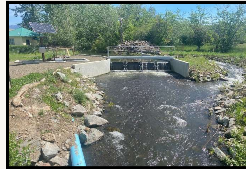
LC6 Diversion after construction
