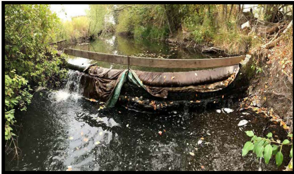
Israel-Ames Diversion (LC6) prior to construction
